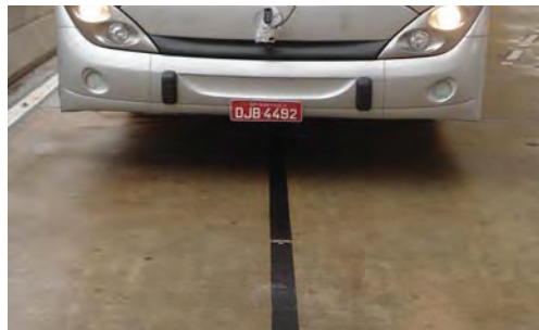
FIGURE 4 - Lane Marking painted on the busway (lane width: 100 mm) - Sao Paulo City's BRT - Espresso Tiradentes.
